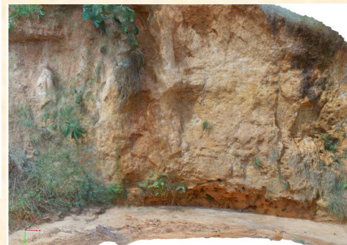
Toe-slope erosion along gully channel
